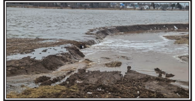
The valiant efforts to create a dyke to protect the building saw it overcome and the lowest end. Lawrence R Nicoll photo.
