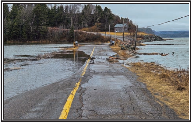
The tides were even higher on March 11, Spencer’s Island waterfront took a real hit, the beach road and the bypass were all flooded. Hopefully the RV site did not receive too much damage. Lawrence R Nicoll photos.
