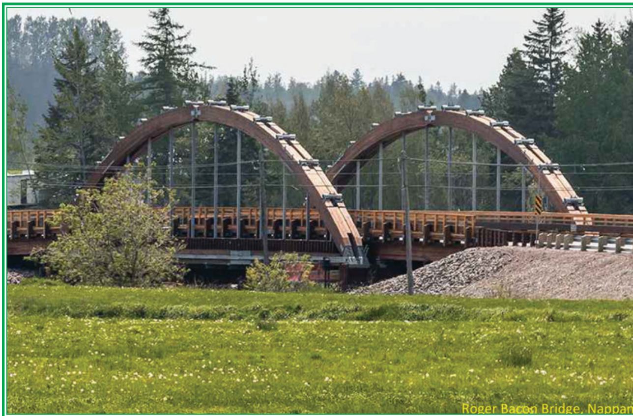
The tender is out and closes on April 6th. To be constructed of wood similar to the Roger Bacon Bridge in Nappan, inside sources indicate the bridge has already been ordered. New Bridge to be Treated Glue Laminated Timber.
