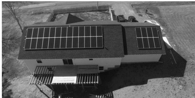
Drones are used to provide an overall aerial view of a solar panel installation. This group of photos show installations completed by Renewly Solar on Colchester County. (Submitted)
